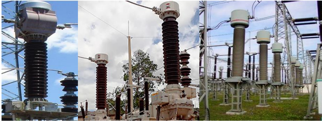
Fig.5.10 Voltage transformer
