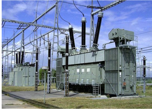
Fig.5.7 Power transformers
