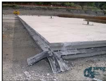
Figure 04 : Joint de construction
